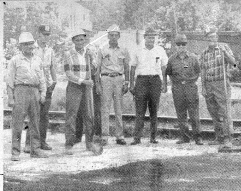
CROSSING REPAIRED — Shown above are City of Iuka workmen and Frederick Construction Co., who repaired two of the railroad crossings in Downtown Iuka last week. Fred-
